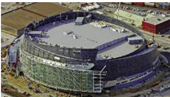
Bank of Oklahoma (BOK) Center, Tulsa, Okla. 220,000 square feet of JM PVC-60 Roofing Contractor: Oklahoma Roofing & Sheet Metal Inc., Oklahoma City, Okla. Owner: City of Tulsa
